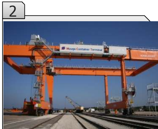
RMGC (Rail Mounted Gantry Crane)
